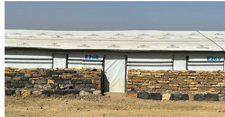
Temporary shelter with fortification. ©Sophie Gebreyes/LWF. Seba Kare. May 2022
