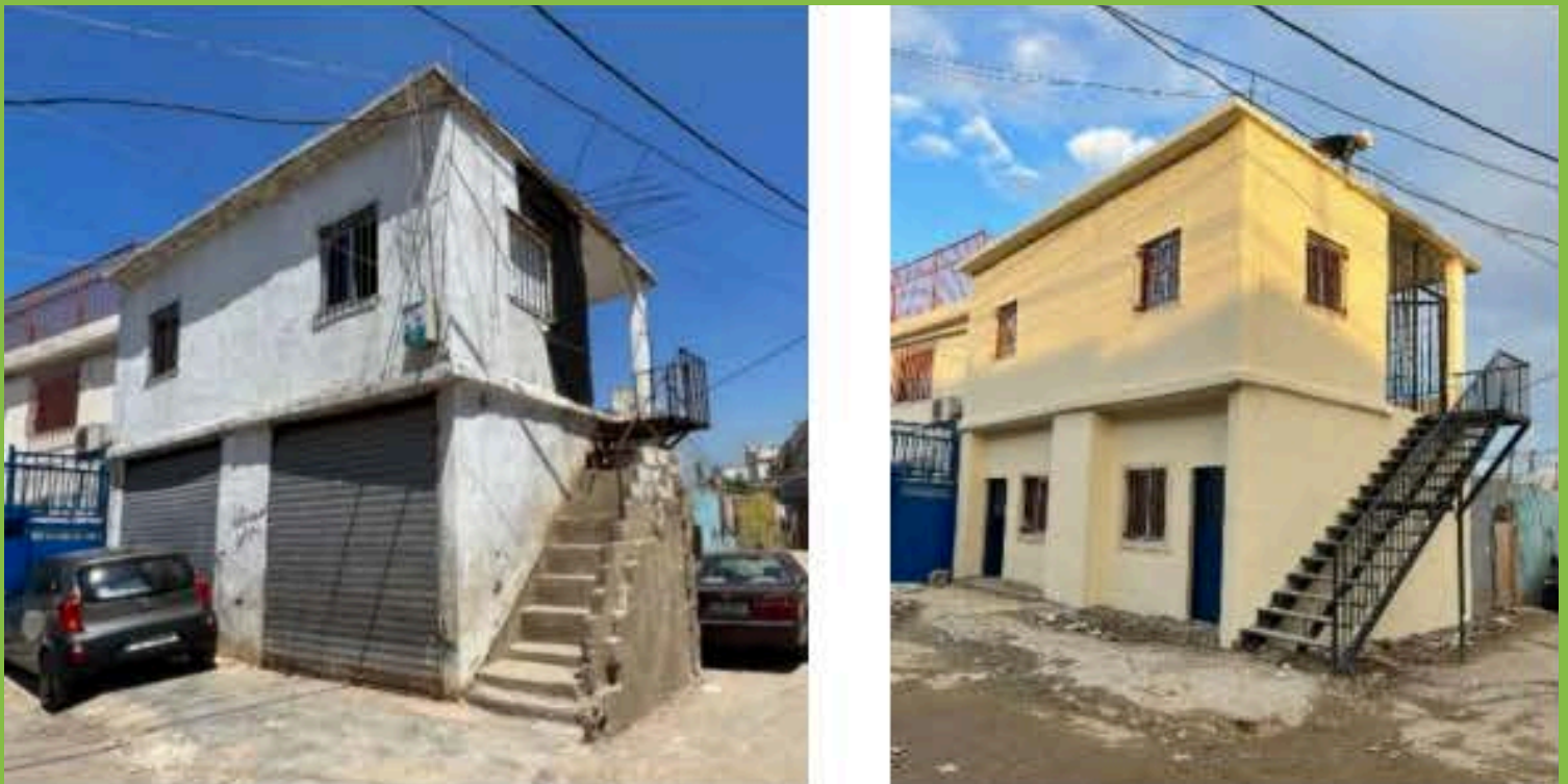
Photo shows the pre and post rehabilitation of the Tahaddi vocational training center in Lebanon supported by LWF.
