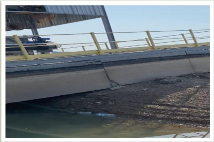
Figure 17: Breaking the intakes and unscrewing the pipes in the Faida water
