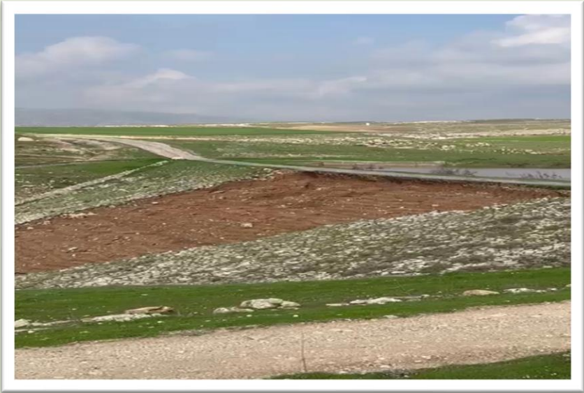
Figure 22: An earthen dam damaged by floods in a single season
