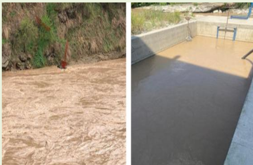
Figure 18: Breaking the intakes and unscrewing the pipes in the Faida water
