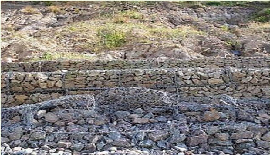
Figure 28: Gabion structures in a mountain area.
