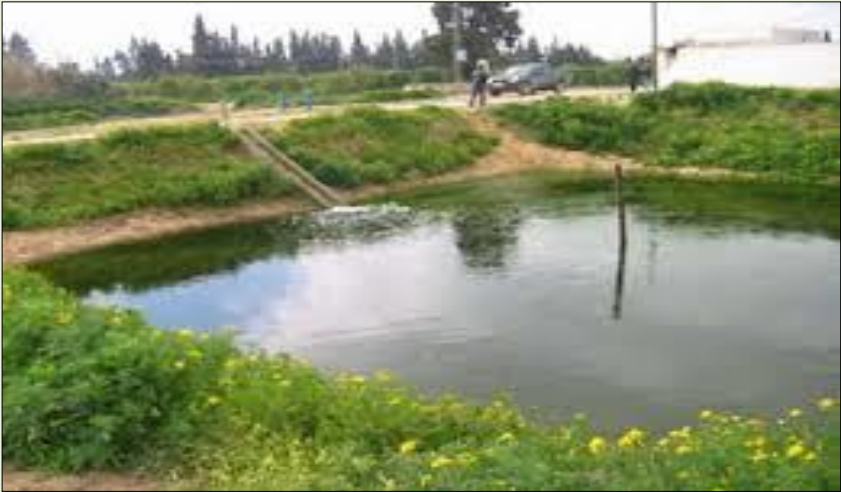
Figure 30: Small basins and open channels to store and harvest water.
